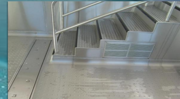
Public stairs (incl. Step marking and handrail)
